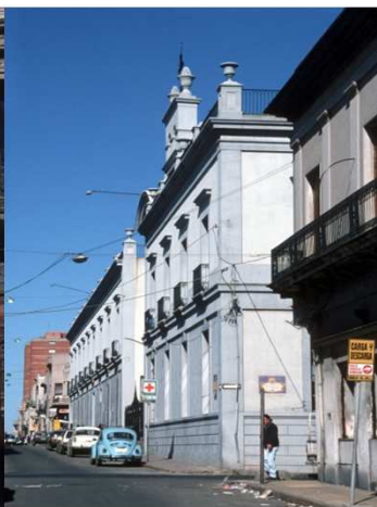
4. Hospital Maciel SMA-S073-004
