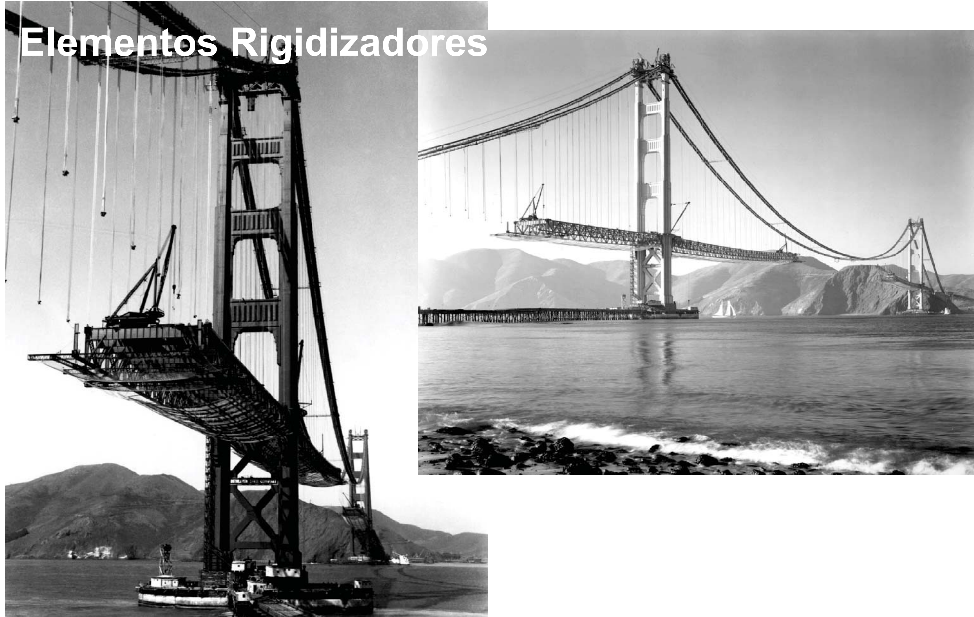
Proyecto: Golden Gate Bridge [1937] Strauss-Morrow-Ammann
