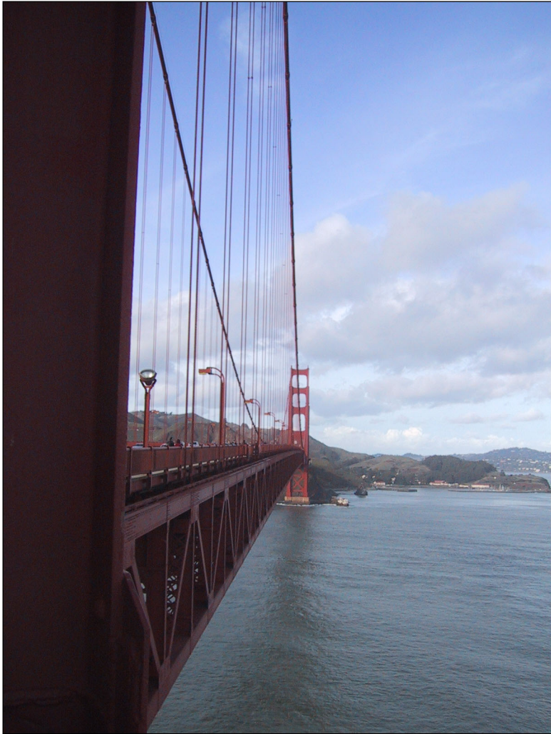
Golden Gate Bridge, San Francisco, California
